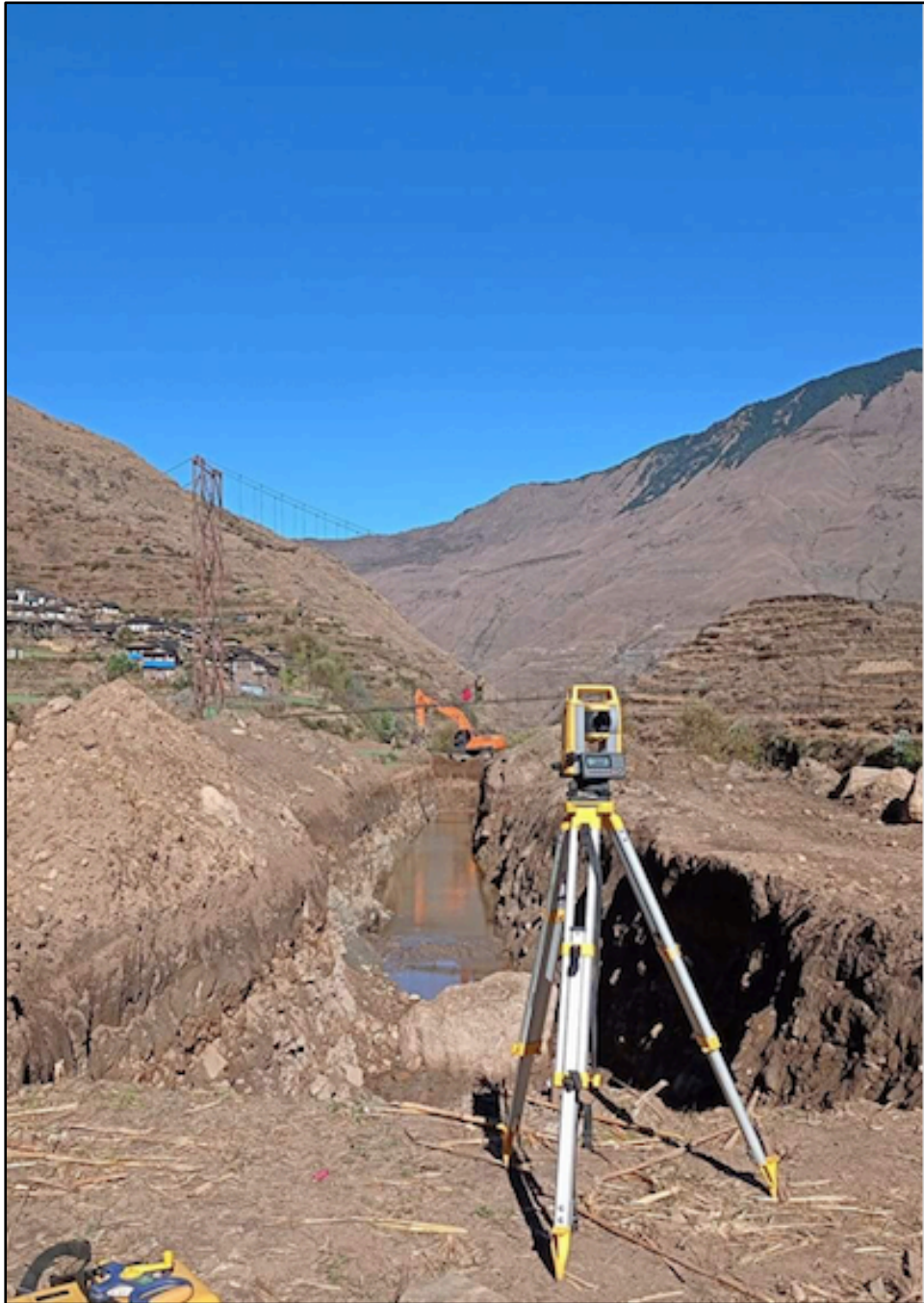
Approach Canal Excavation of the 998kW Saniveri MHP, Rukum East
